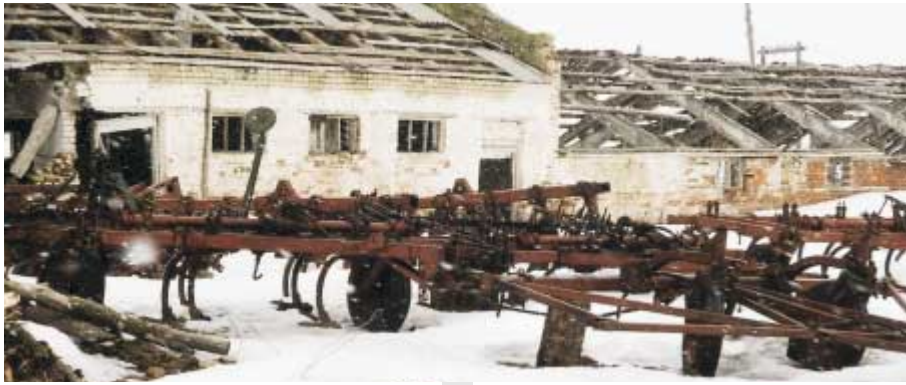
Many Russian buildings are in a poor state of repair...
